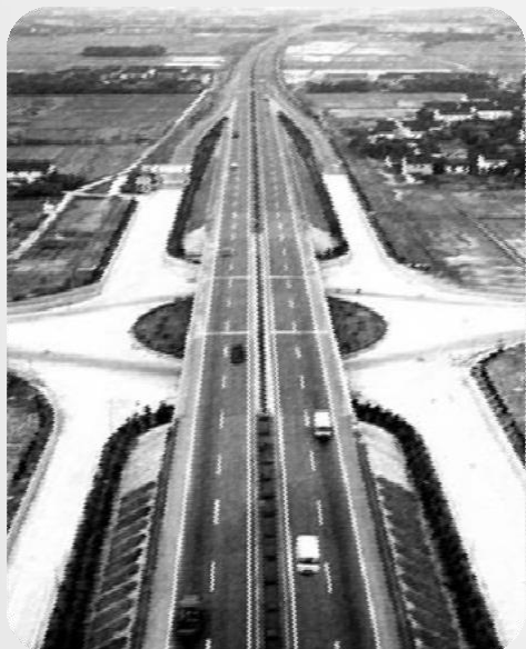
Shanghai—Jiading Expressway (28 km)
