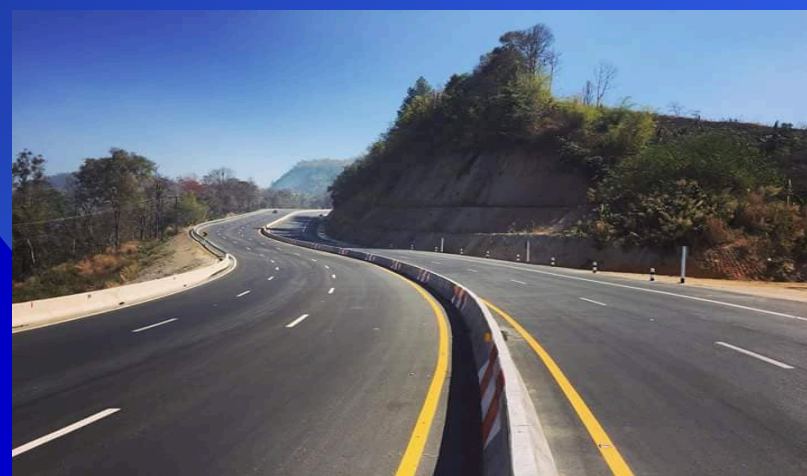
Photos: Department of Highways
