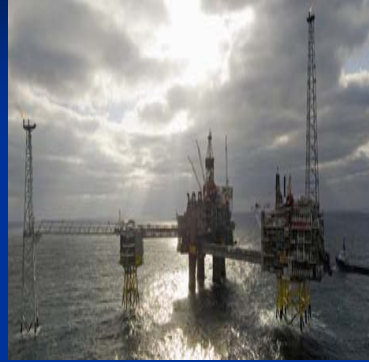
Sleipner CCS Project
