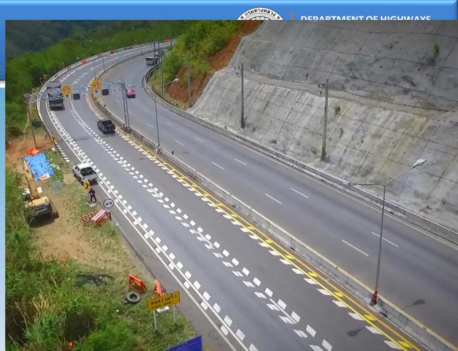
**Optical speed bar : Speed reduction**
