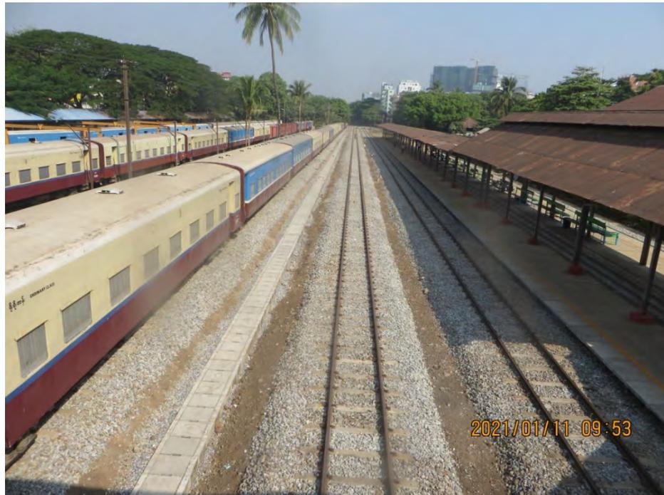
**Note : Pre Final inspection for track profile are completed and Final manual rectification to close out the Track Geometry (Level and Alignment) are in progress.**
