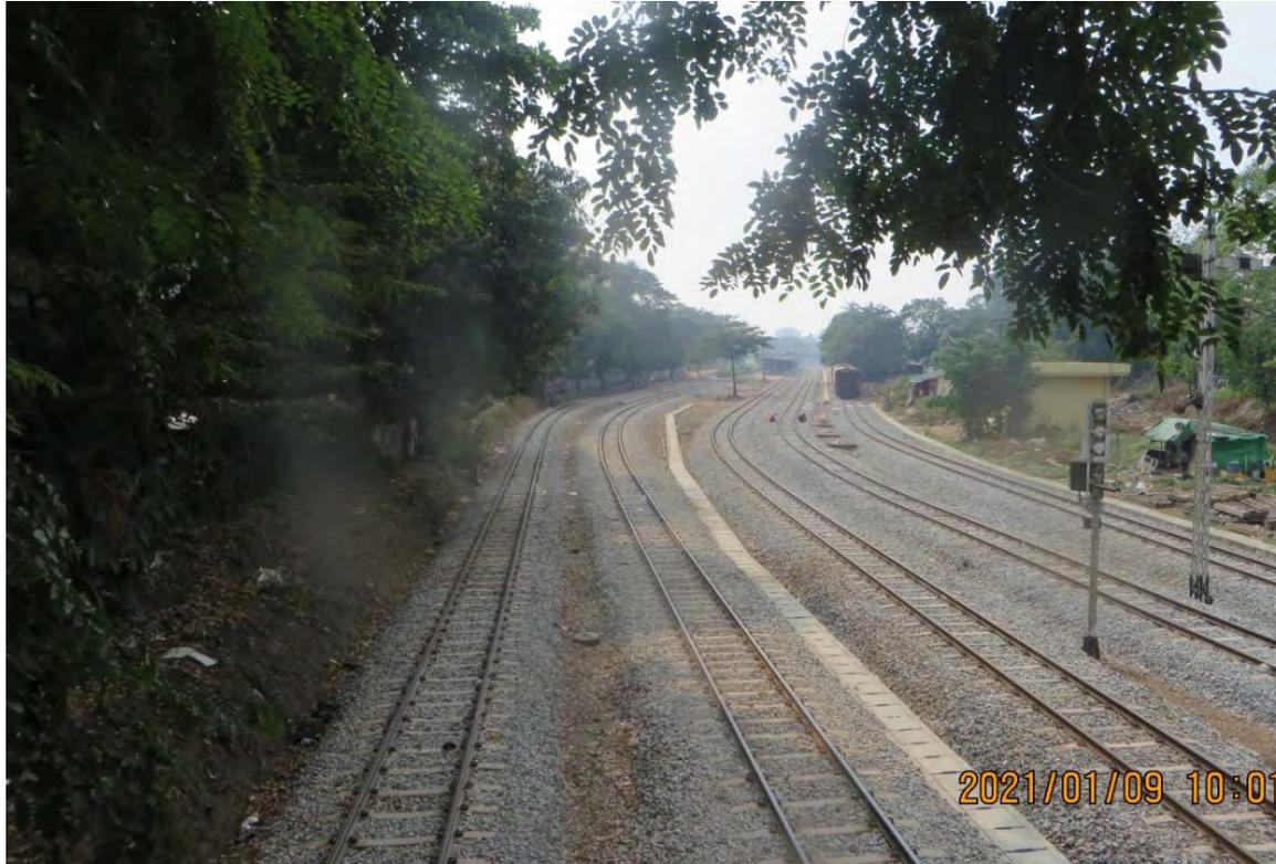
**Note : Pre Final inspection for track profile are completed and Final manual rectification to close out the Track Geometry (Level and Alignment) are in progress.**
