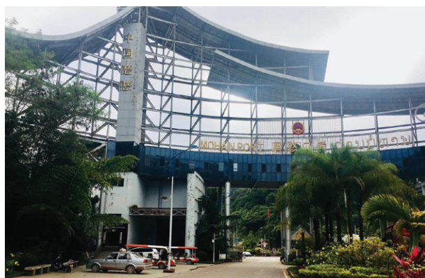
Mohan Border Crossing Facilities. China Customs building in Mohan at the Lao PDR-PRC border. Photo credit: Li Guoliang
