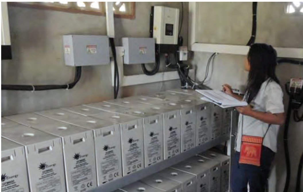
Inspection of the batteries in the powerhouse
