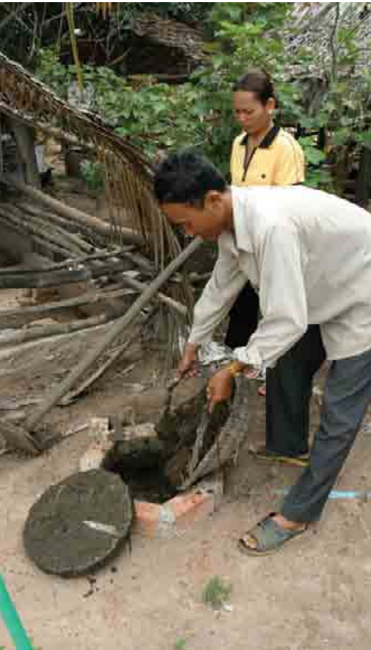
■ Emptying waste into a household biogas collector, also known as an anaerobic digester, Cambodia.
