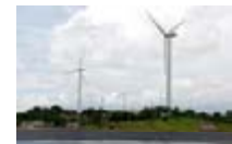
Lam Takong Dam 18.0 MW
