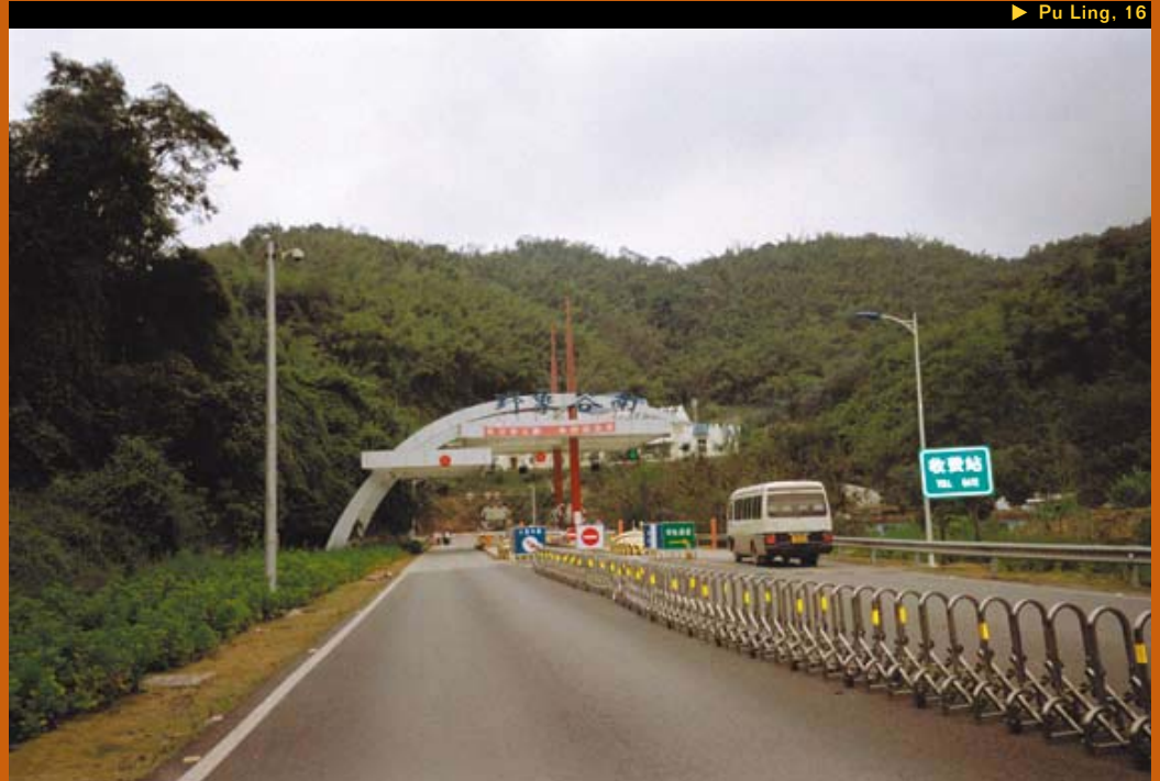
► Toll gate on the Kunming-Bangkok Highway (PRC). ▼ Scene at the Lao Bao border gate. It shows Lao Bao's development (Viet Nam).
