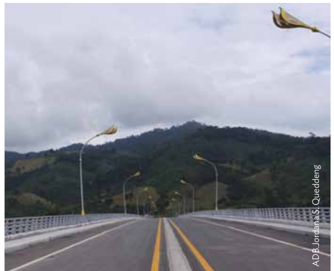
The Fourth Thai–Lao Friendship Bridge is 630 meters long with a span of 480 meters and is 14.7 meters wide. It is located about 10 kilometers from Amphoe in Chiang Kong in the northeastern part of Chiang Rai in northern Thailand and about 12 kilometers from Ban Houayxay, the capital of Bokeo province in northwestern Laos
